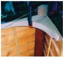
Above: Interior joinery started with the breasthook and quarter knees. Below: The combined width of the rubbing strake, gunwale, sheer plank, timbers and inwale came to 3" (75mm), so 4" (100mm) copper nails and roves were needed to rivet all these layers together.
